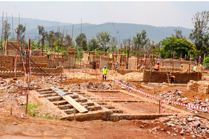
Groundbreaking Celebration attendees walking about the Leadership Center construction site
